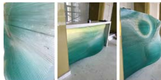
These pictures of the reception desk during its assembly show 116 uniquely shaped glass pieces stacked to form an undulating 3d surface.
