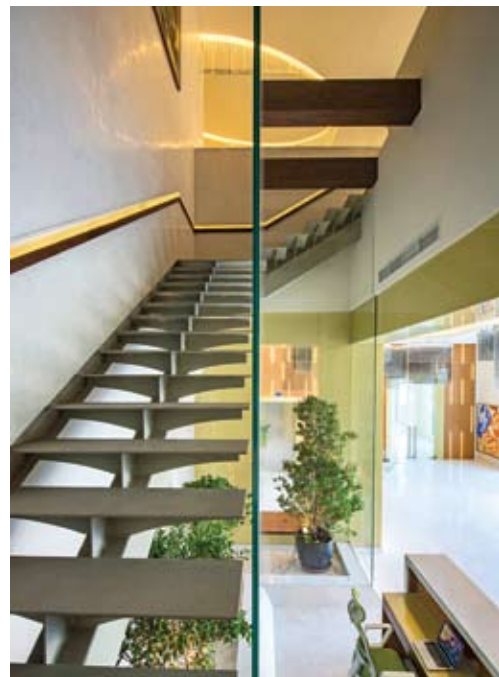
The cantilevered MS staircase leading from ground to first floor is contained behind the 6m tall frameless glass.
