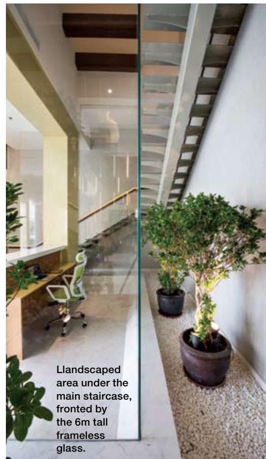
The cantilevered MS staircase leading from ground to first floor is contained behind the 6m tall frameless glass.
